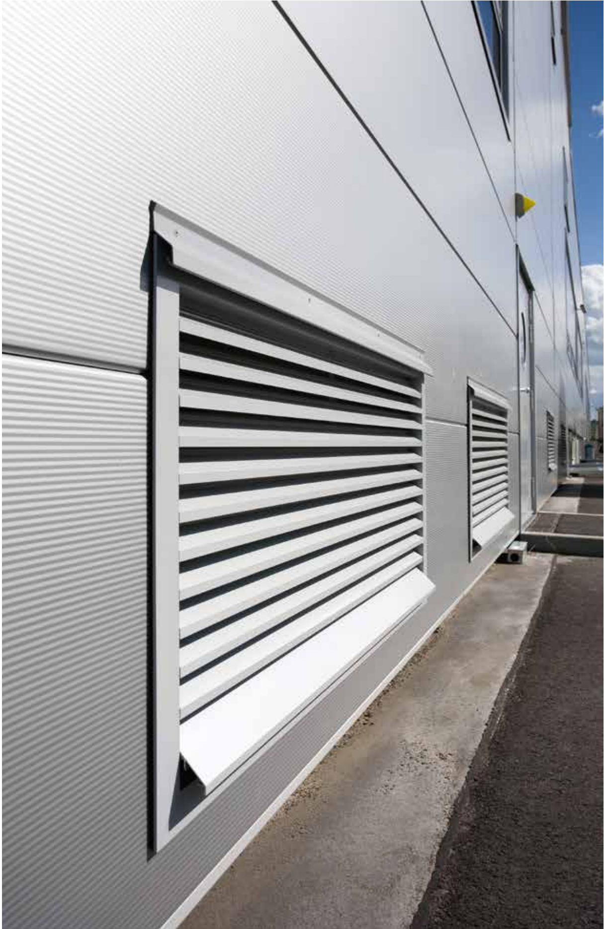
Built-in wall louvre, heavy-duty series 481 (see p. 50)
